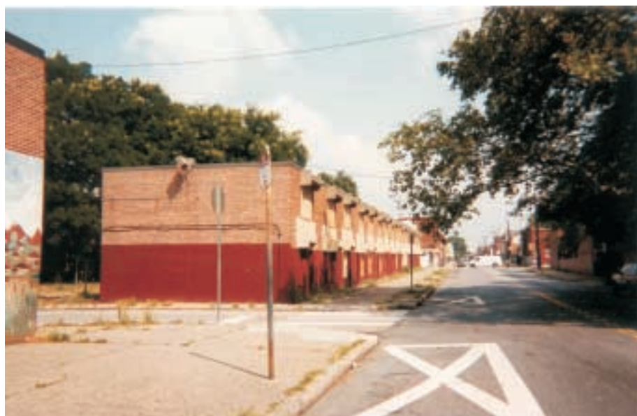
Severely deteriorated developments have been slated for demolition and reconstruction.
