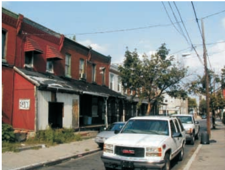
PHA has the difficult task of managing severely deteriorated scattered sites units.
