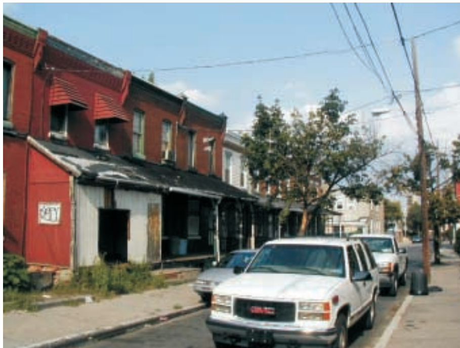
PHA has the difficult task of managing severely deteriorated scattered sites units.
