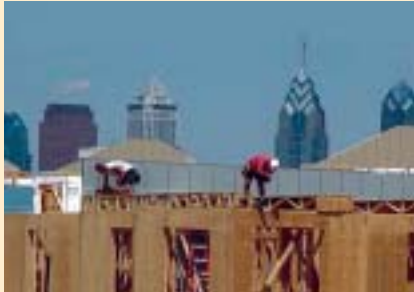
Tasker Homes Construction– South Philadelphia
